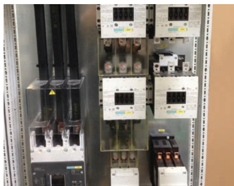
Application pictures: Flexibar directly connected on MCCB's front access connection.
