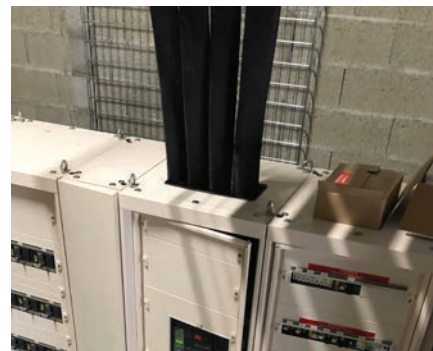
Example of global cut out on magnetic plate (steel)
